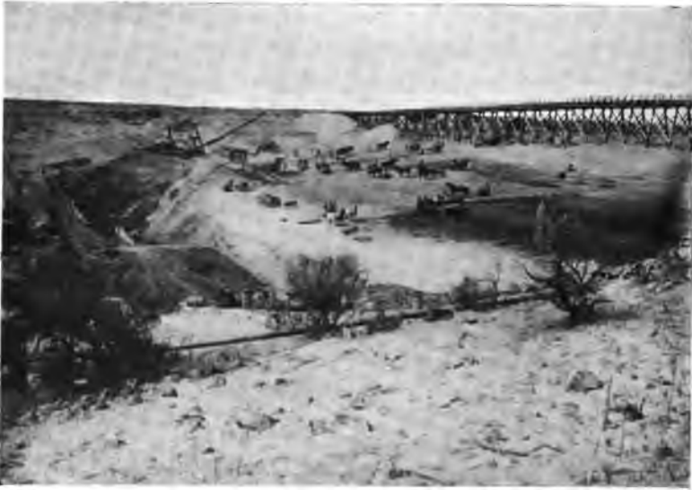
FIG. 204.—Cold Springs Dam under Construction, Umatilla Valley, Oregon.
